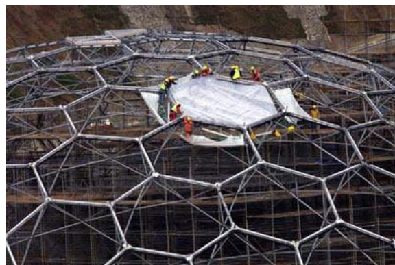
Fig. 12: Each ETFE pillow is secured in the steel framework.
